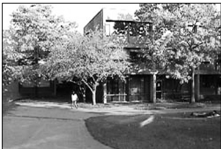
The dorms new to energy challenges (top to bottom: South, Carnegie, Keehn, and Root Residence Halls.)
